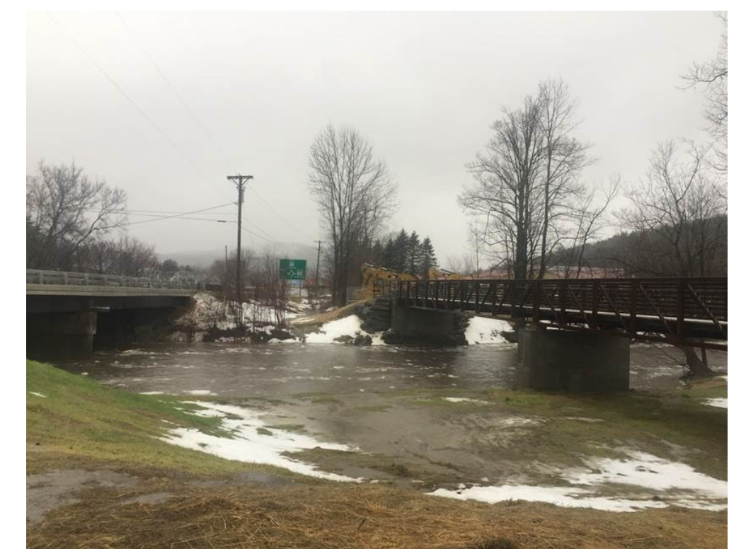
January 12, 2018 Post-Construction Flooding
