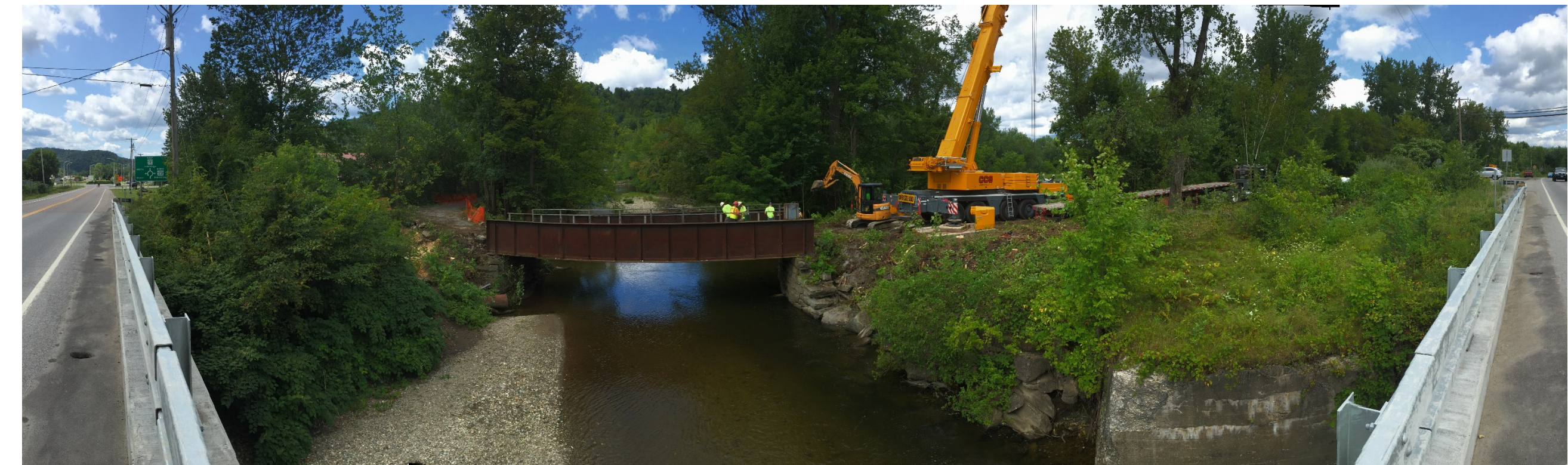
August 23, 2017 Start of Construction
